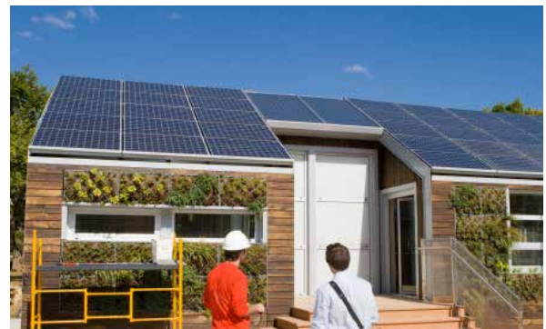
Ensuring comfort and maximizing energy efficiency are both key concepts of the HERS rating
